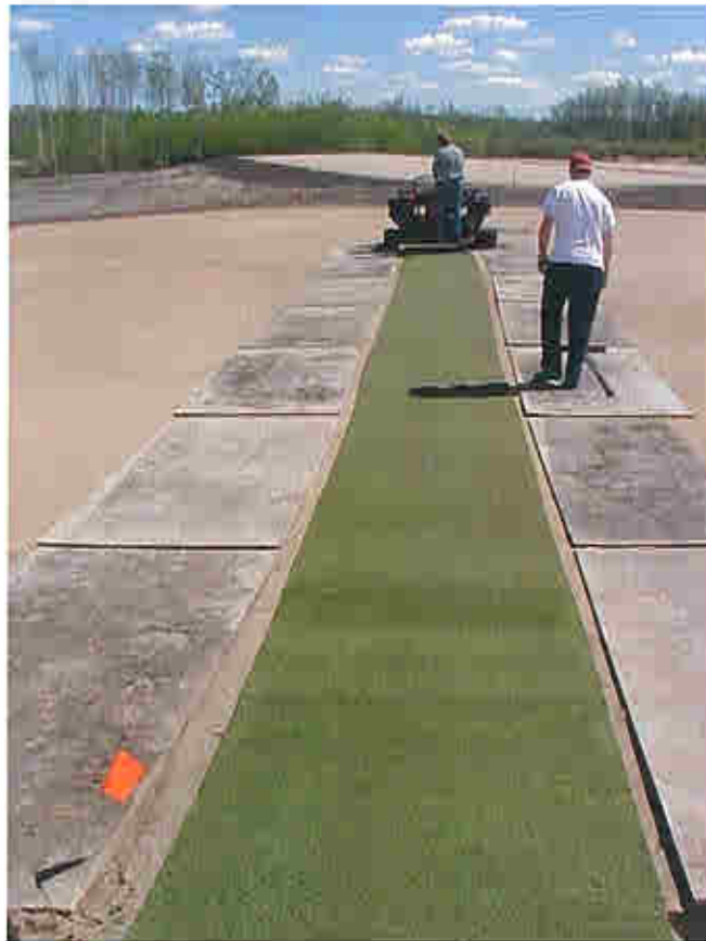
Laying the big rolls.
