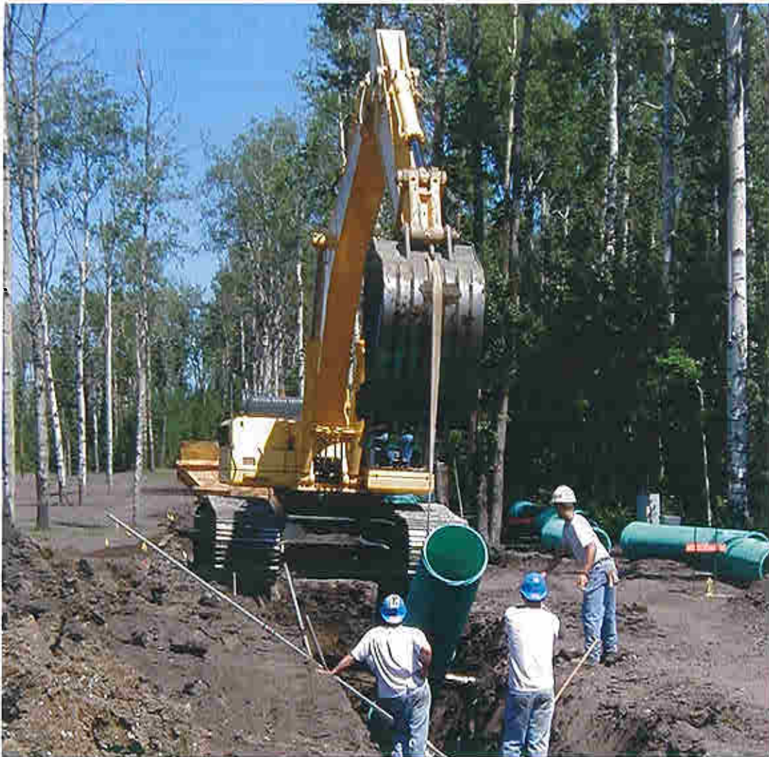
Installing the main irrigation line.
