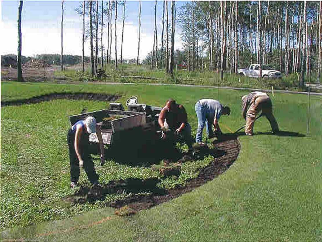
Cutting out the bunker.
